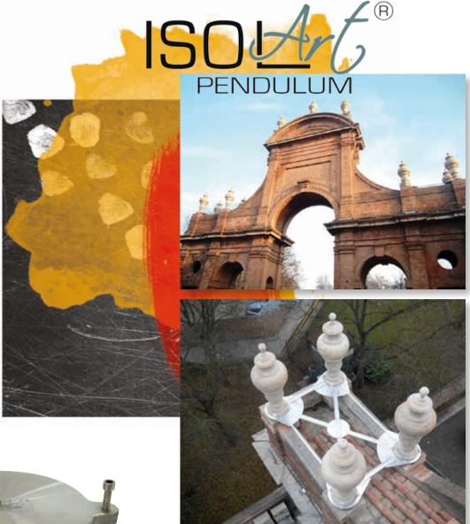
ISOLART® PENDULUM has recently been employed for the seismic protection of the Bust of Francesco I d'Este by Gian Lorenzo Bernini in the Estense Gallery in Modena, Italy, and for the protection of the pinnacles of a three-arched masonry city gate, in Ferrara, Italy (Picture above).
